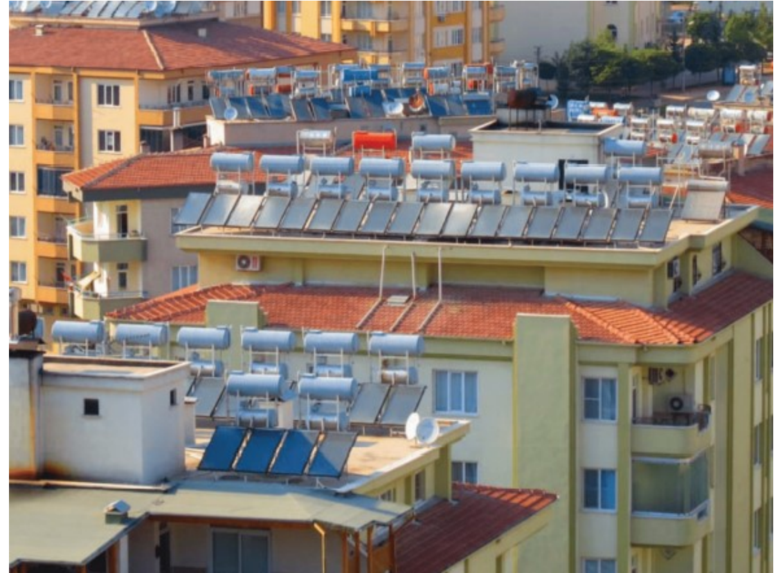
Figure 4-1 Solar water collectors on the roof of residential buildings.
